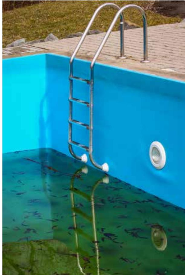
If a swimming pool or hot tub has flooded or received large amounts of silt and trash and the water is muddy, remove the trash, then attach a sump pump, and pump the water out directly to the sewer. (Do not drain pool by back washing the filter.)
